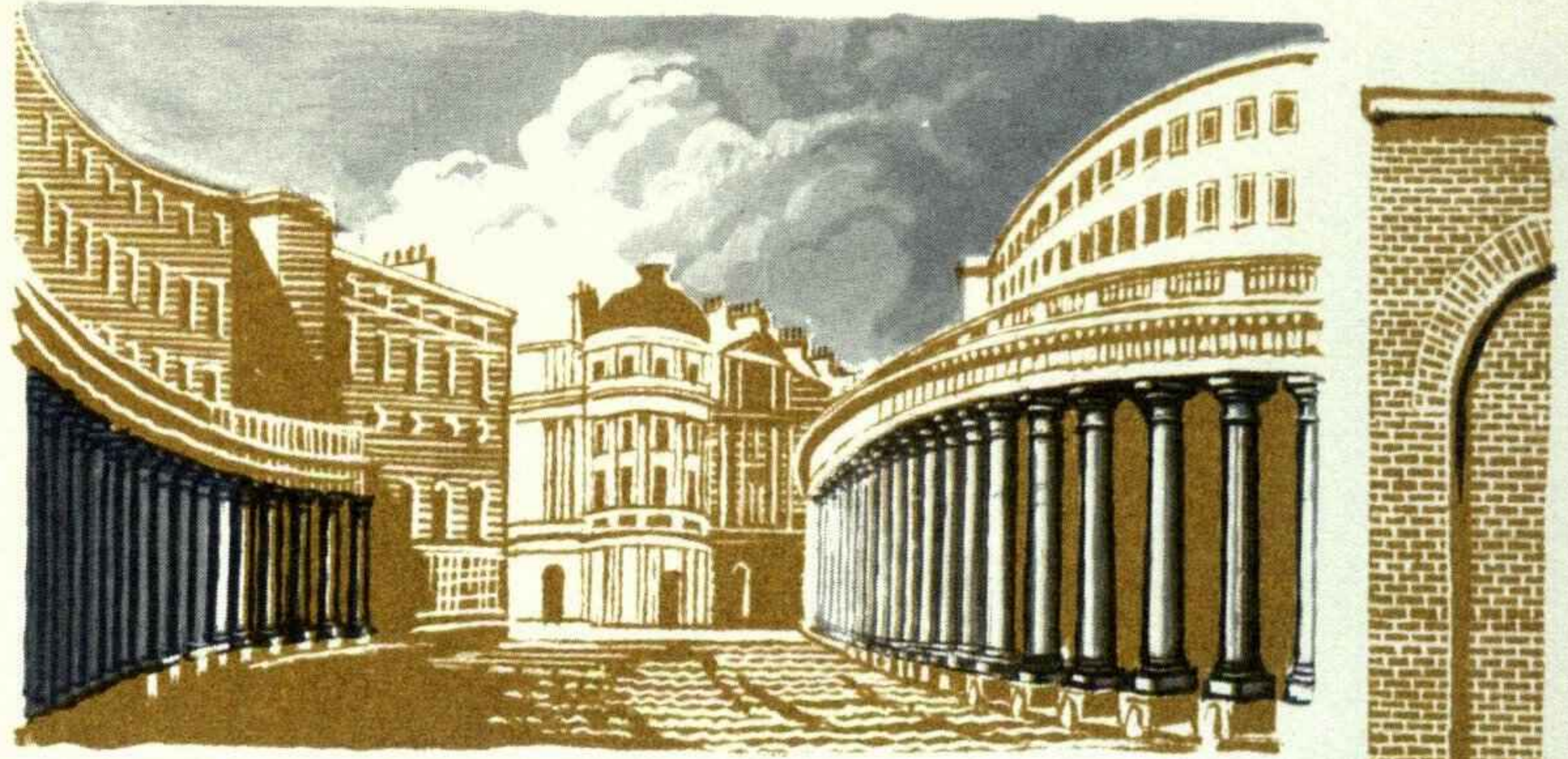
A The Quadrant, Regent Street 1818 Cast-iron columns
